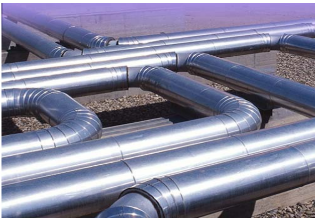
The computer models created by Greg Perkins from UNSW on ac3 's computers enables companies to determine the economic viability of underground coal 'gasification'.
