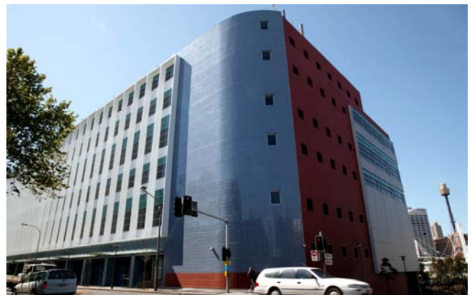
Global Switch's data centre at Ultimo on the outskirts of the Sydney CBD is Australia's largest carrier-neutral data centre.
